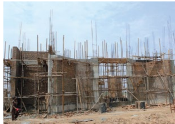
OVERSEAS BLOCK-C (SECTOR MOSQUE) BRICK MASONRY IN PROGRESS
