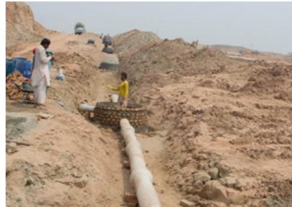
OVERSEAS BLOCK-A (LANE #1) CONSTRUCTION OF MAIN HOLES
