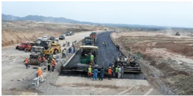
ASPHALT WORK AT MAIN ROAD BETWEEN OVERSEAS BLOCK & GENERAL BLOCKS
