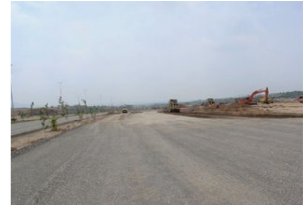
OVERSEAS BLOCK-C (COMMERCIAL ROAD) SUB-BASE IN PROGRESS
