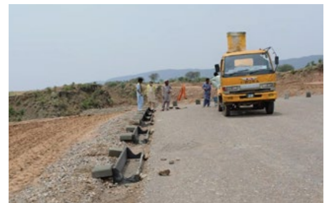
ACCESS 1 (1+800 ~ 2+700) SAUCER DRAIN IN PROGRESS
