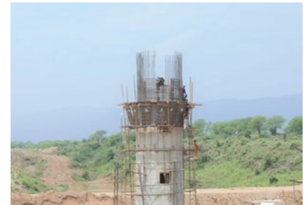
OVERSEAS BLOCK-C (OHWT) REBAR FIXING FOR SHAFT IN PROGRESS
