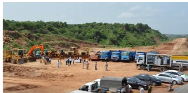
A NEW CREW OF HEAVY MACHINERY
